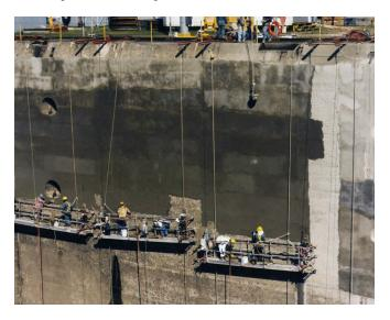
The culverts' rehabilitation process included cleaning the walls by water blasting to remove loose materials and prepare the surface. A shotcrete application using 17,237 kPa (2,500 psi) mortar with 3% Xypex Admix C-2000 per bag of cement was then applied, covering an area of 60,000 m² (645,834.63 ft2). The thickness of the mortar cover varied between 1.25 cm and 3.85 cm (1/2 in to 1 in). In total, over 54,400 kg (120,000 lbs) of Xypex Admix C-2000 were used.
